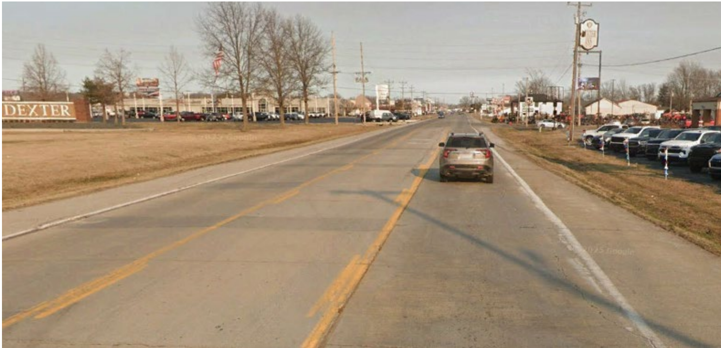
Figure 66: Central Dexter – Typical Conditions on BUS 60 (CD.1)
