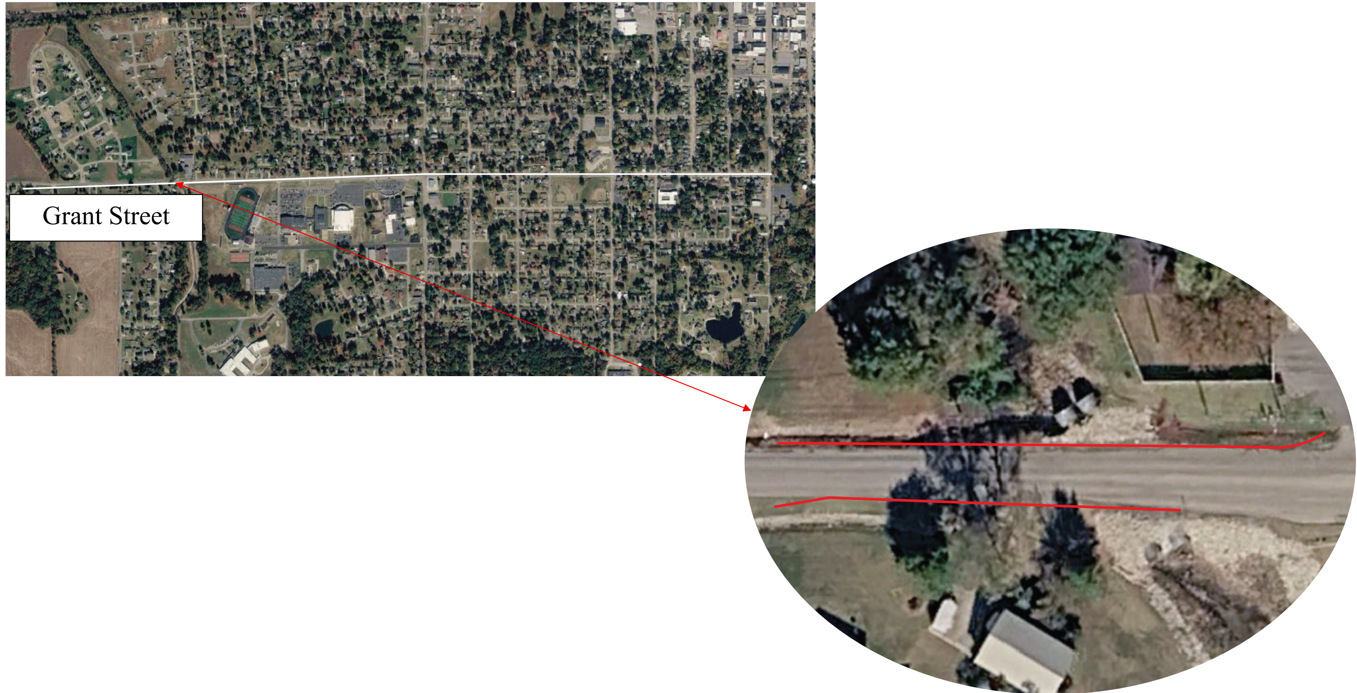
Figure 51: Roadside Protection Improvement – Grant Street
