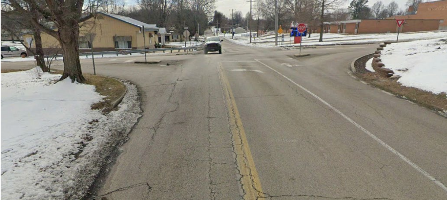
Figure 74: One Mile Rd. SD.3 (2 of 3) Intersection with Grant St.
