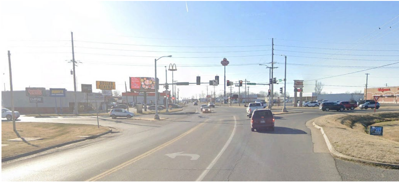
Figure 65: Central Dexter – BUS 60 / One Mile Road Intersection (CD.1)
